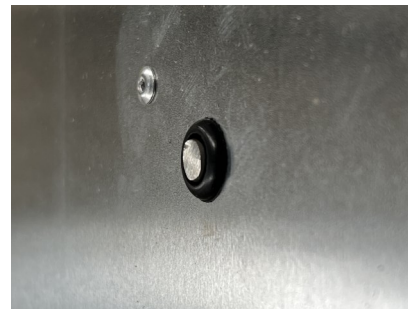
Lateral Bolt rests on Tee Grid during filter change
